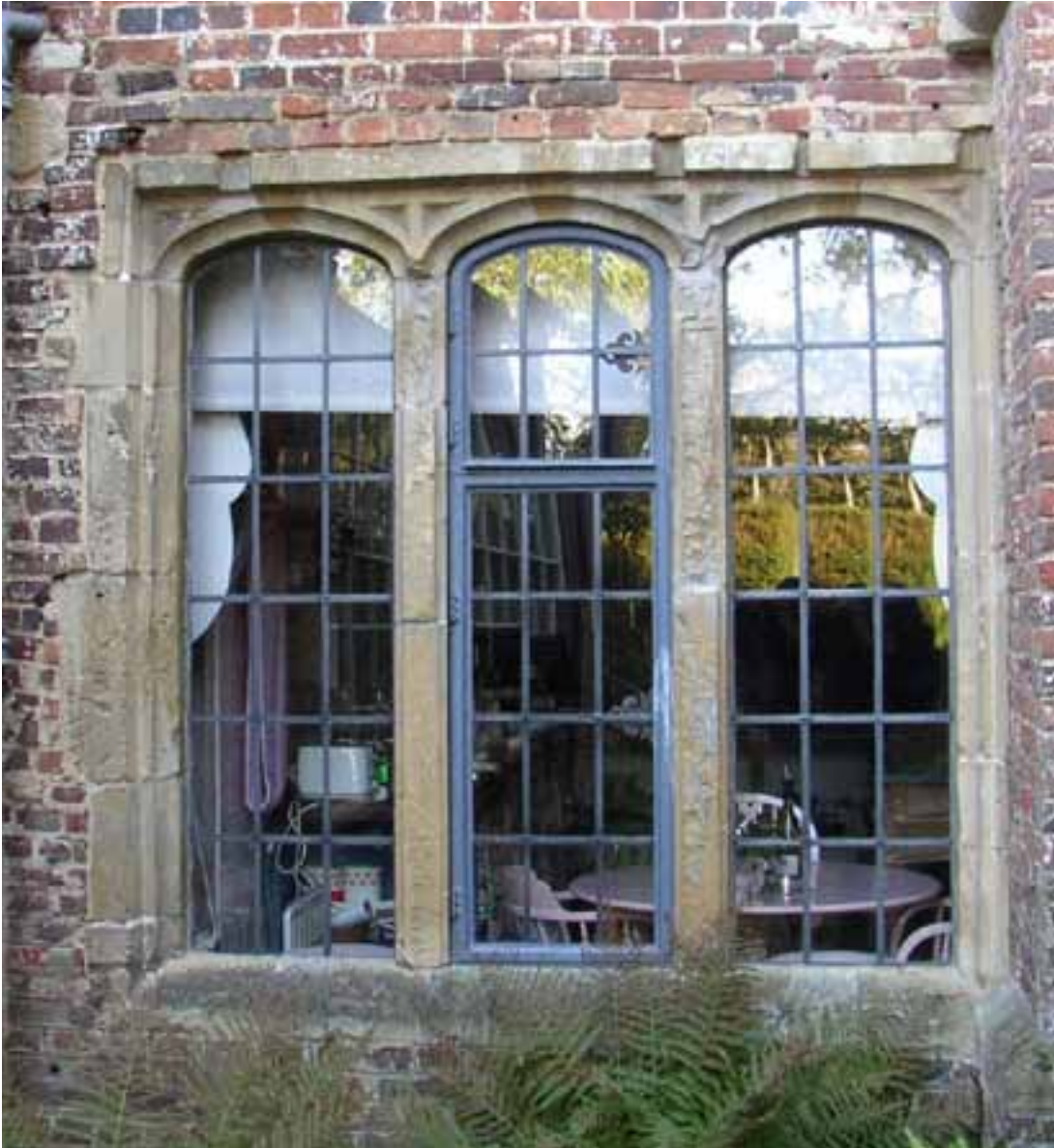
05 Leaded light windows can be difficult to make draught free and secondary glazing might need to be considered. © Oxley Conservation
