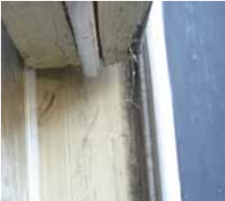
09 Brush pile seals added to a sash window © English Heritage/David Pickles
