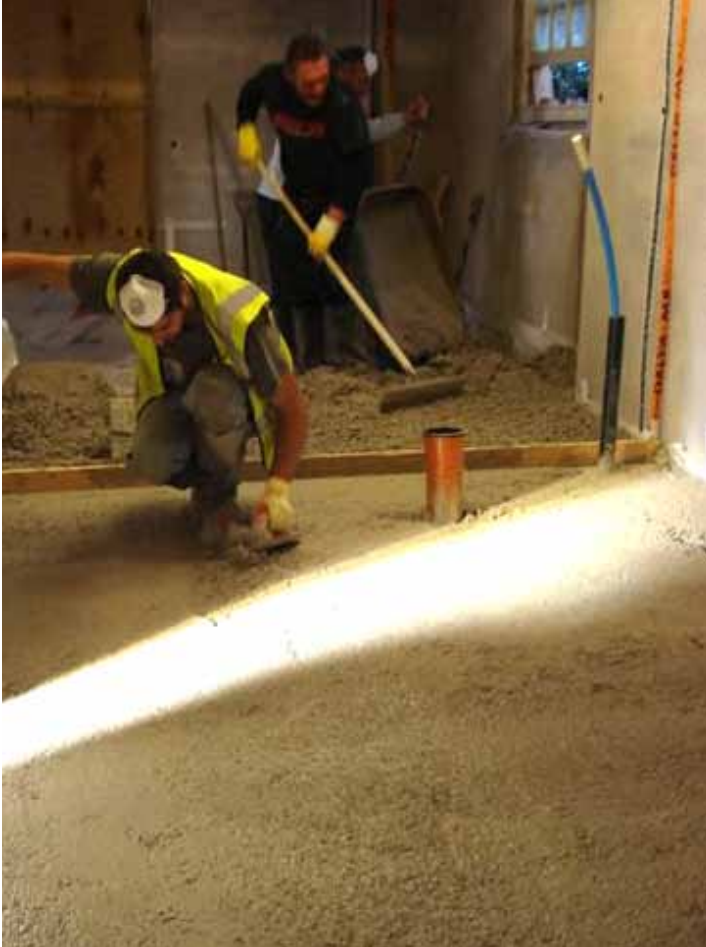
07 A hydraulic lime floor being laid © The Limecrete Company
